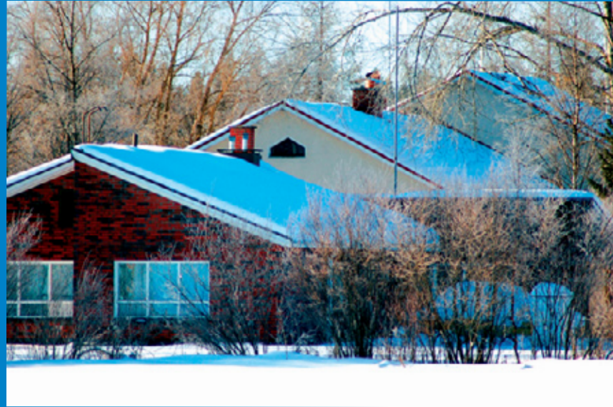
A reception centre in Ruukki, Northern-Finland. Photo: Tuomo Heikkinen
